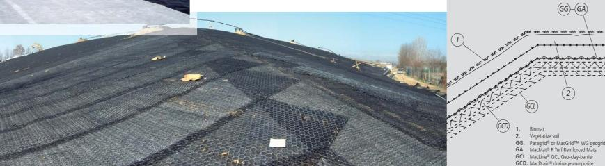
GG. MacGrid<sup>™</sup> WG or Paragrid<sup>®</sup> GCD. MacDrain<sup>®</sup> Drainage geocomposit GCL. MacLine<sup>®</sup> GCL Geo-clay-barrier GA. MacMat<sup>®</sup> R Turf Reinforced Mats
