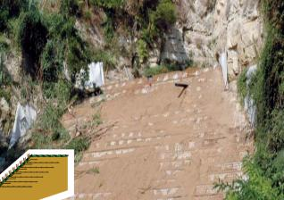
MacGrid™ WG are often also used in combination with bioengineering techniques in order to provide the structural strength combined with an environmental
